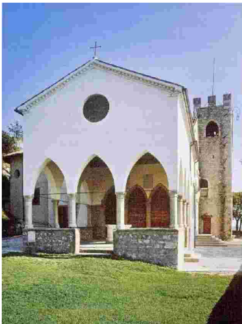
Saint Augusta's sanctuary. Loggia opposite the old entrance of the sanctuary, erected on the occasion of the expansion works (1450 – 1452).
